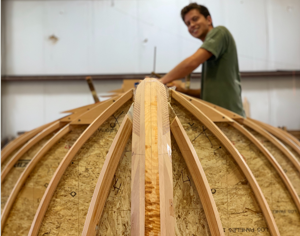
Arey's Pond Boatbuilder, Dustin Page, works on the hull of a 23' custom catboat. The hull and brand new Yanmar engine are now for sale on our brokerage site. Learn more here.
